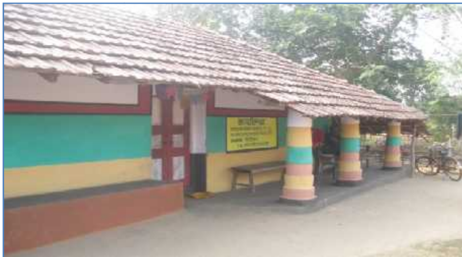
Clean and smooth walls with organic colour on it are symbolic of a Santal house ( Buruj Khunti) in Dumuria
