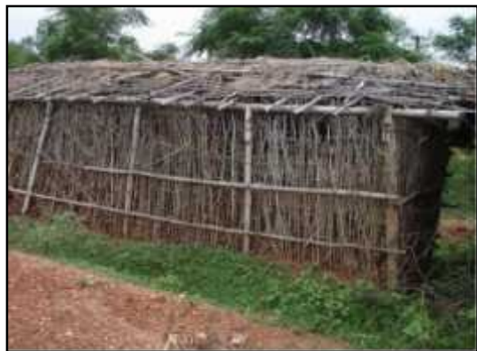
Jhanti : Dudhchuwa, Dhalbhumghar Block
