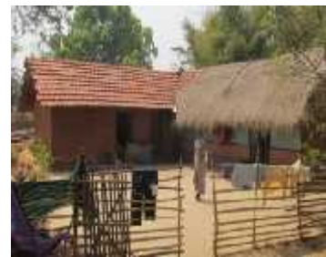
Nuniya: Dumariya block Tile and Hay Construction
