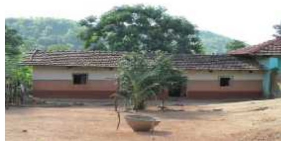
Buruj-Khunti housing with Tiles roof
