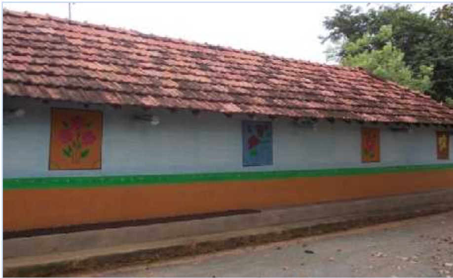
Walls painted with natural colours, designs of flower etc. (site: Pindrabera, Gamharia block)
