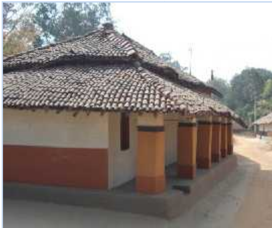
Roofs of Aat Chaala house, Patharbhanga, Potka Block
