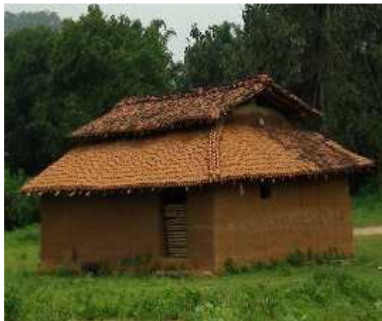
Roofs of Chha Chaala house, Dumuria Block
